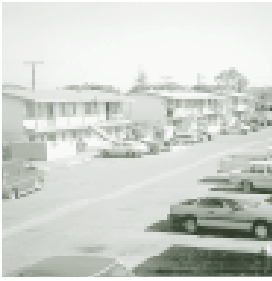
Deteriorating and overcrowded apartments in North Orange County.
