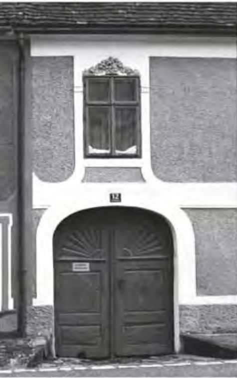
significant entry door
