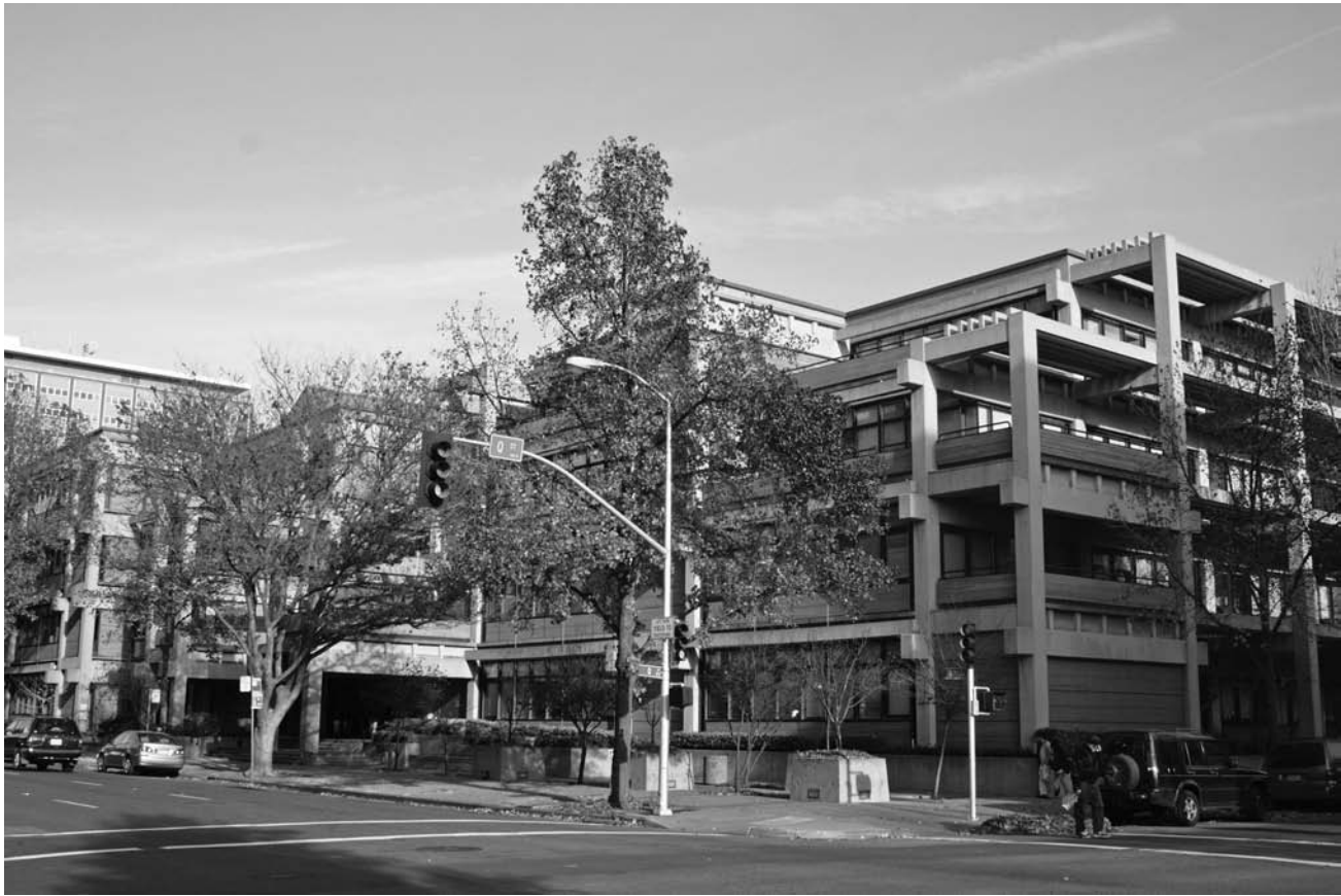
Figure 1 Office of the State Architect, Bateson Building, Sacramento, 1977–81 (author's photo).
