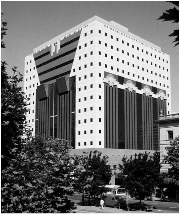
Figure 13 Michael Graves, Portland Building, Portland, Oregon, 1979–82 (photo: Steve Morgan Creative Commons Attribution–ShareAlike 3.0 Unported License).
