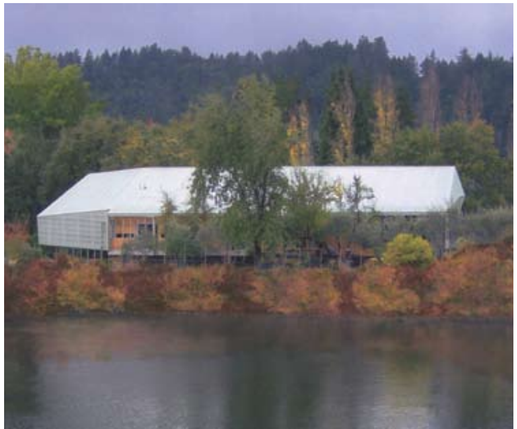
Kuth/Ranieri Architects, Lodi Bunkhouse, St. Helena. Honor Award. Photo by Felipe Villas Boas.
