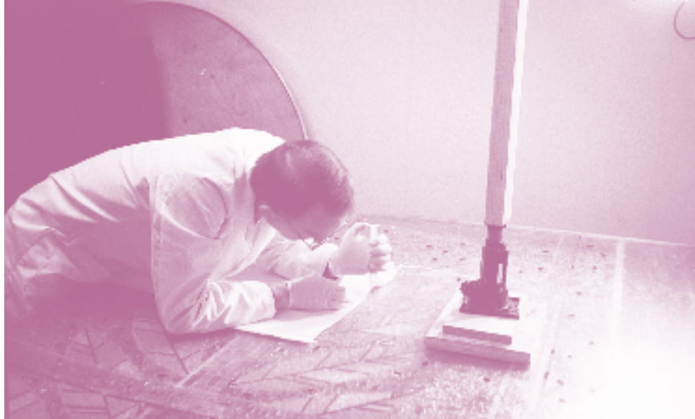
above: Masonic Auditorium mural restoration, injection of adhesive at bowed panel
