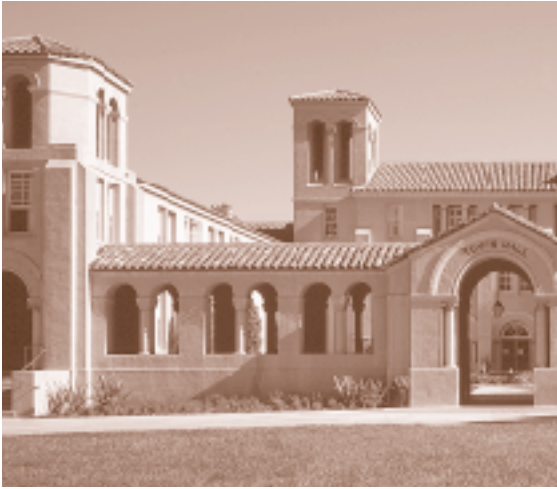
Toyon Hall Renovation, Stanford University // Merit Award
