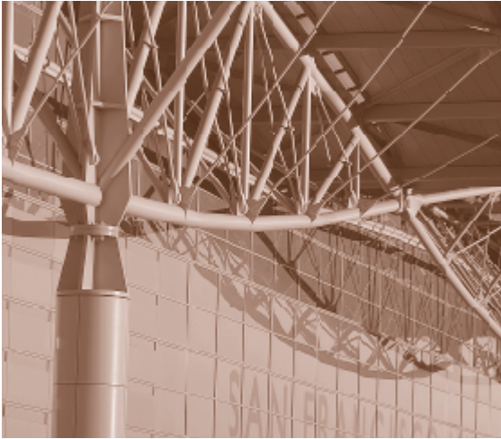
New International Terminal, San Francisco International Airport // Honor Award
