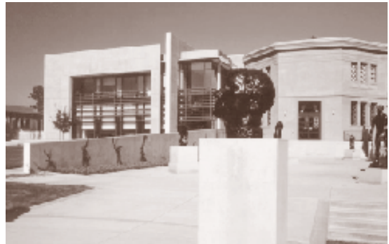
The Cantor Center for the Arts, The Polshek Partnership Architects
