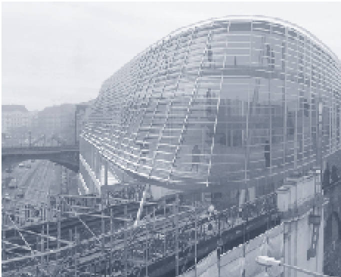
Office Building Spittelau, Vienna 2002-, Silja Tillner Architect.
