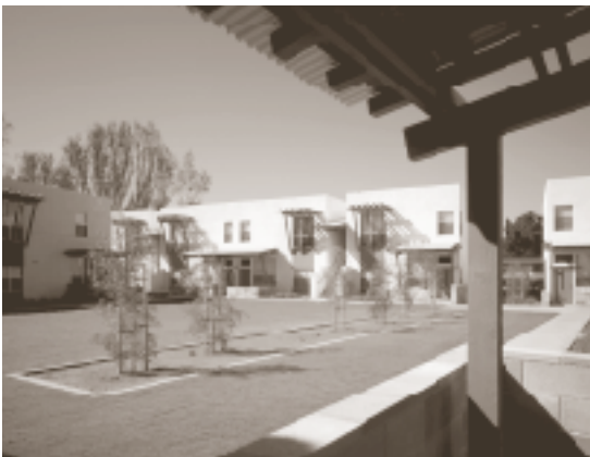
Eucalyptus View Cooperative in Escondido, by Studio E Architects
