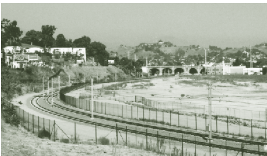
Cornfield Yard, looking north towards Broadway Bridge
