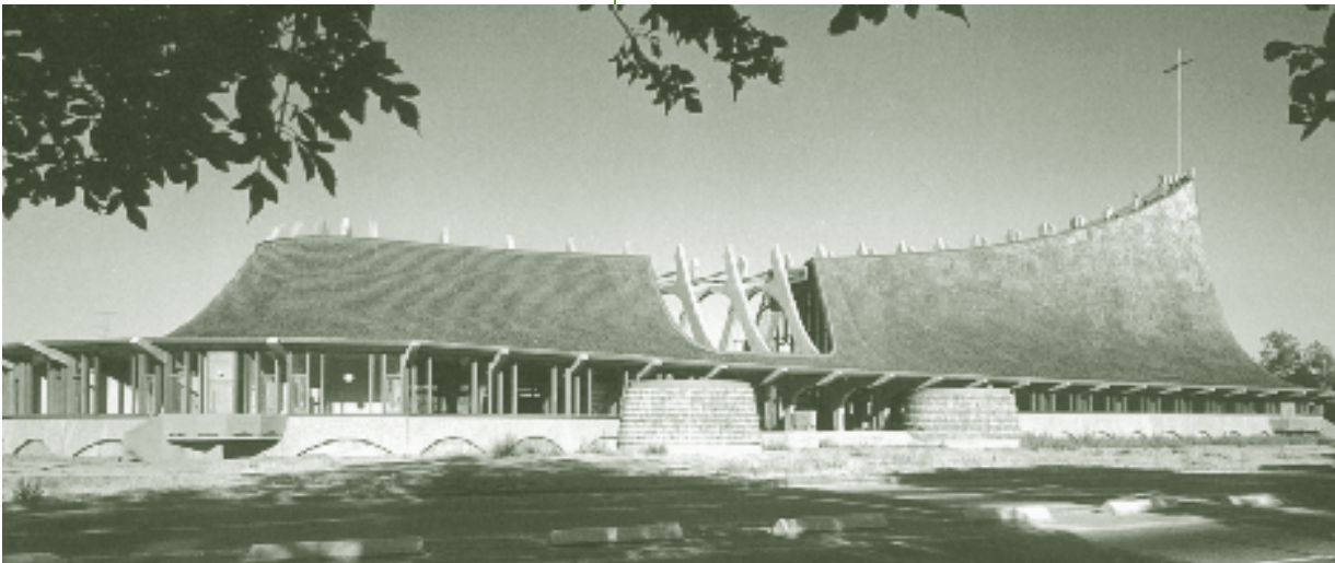
Central Methodist Church, Stockton, California - Continuous concrete bents frame the chapel, community room, and outdoor space.
