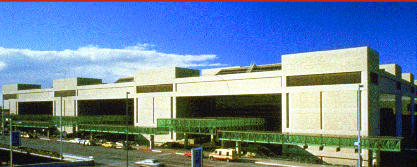
Tom Bradley International Terminal, Los Angeles International Airport
