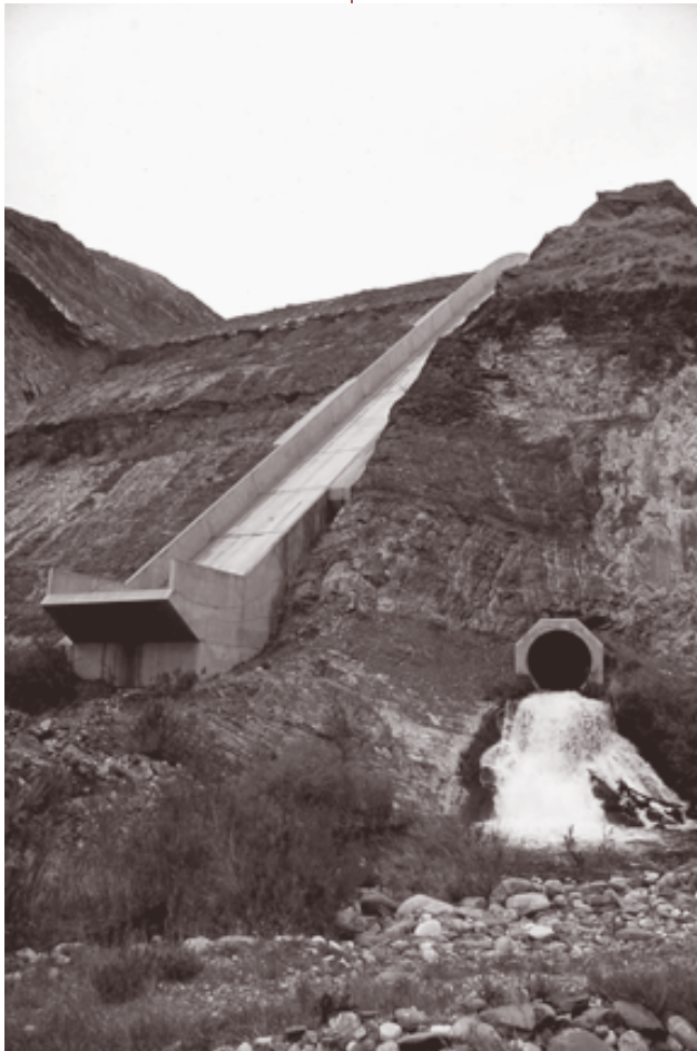
Barton Phelps, FAIA Spillway and Creek Diverter Pyramid Lake Dam
