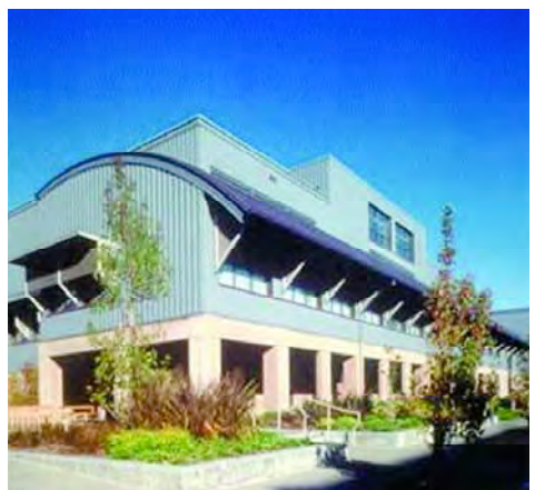
Bayer Corporation, Bio-Technology Campus, Berkeley, California
