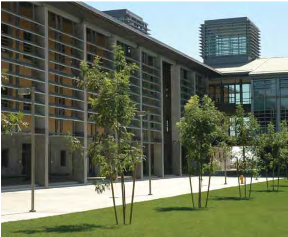
left above: UC Merced Central Plant, Skidmore, Owings & Merrill, LLP, photography by Tim Griffith.
