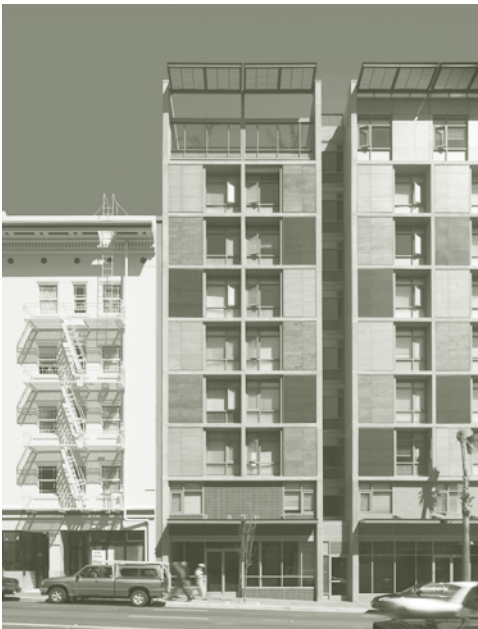
top: Conservatory of Flowers, Golden Gate Park, 1878 (restoration architects, 2003: Architectural Resources Group), photo by David Wakely bottom: Plaza Apartments, Sixth and Howard streets, 2006, Leddy Maytum Stacy Architects and Paulett Taggart Architects, photo by Tim Griffith
