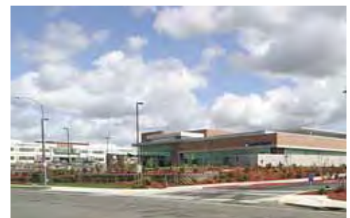
LOBBY AT ENTRY VESTIBULE
