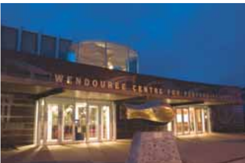
top, phase change spheres; center and bottom, Wendouree Centre for Performing Arts, Ballarat, Victoria, Australia, McIlldowie Partners, photos courtesy McIlldowie Partners and Martin Saunders
