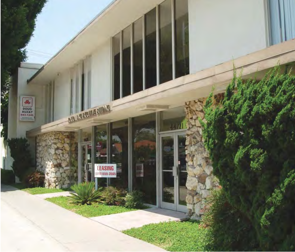
Toluca Lake Executive Building, Marble Architecture, before (left) and after (right).
