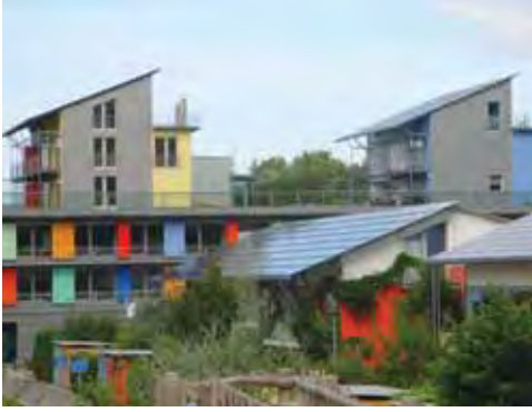
Mixed-Used Plus-Energy-Buildings, Solar City Freiburg, Germany, Architect Rolf Disch. Photo by Thomas Spiegelhalter.
