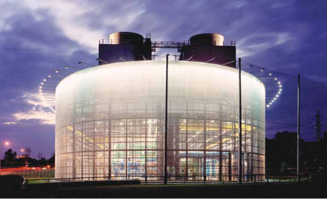
Above: University of Pennsylvania Modular VII Chiller Plant, Philadelphia, Leers Weinzapfel, photo by Peter Aaron/Esto.
