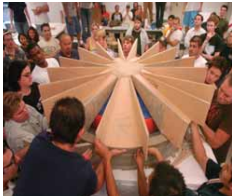
left, Roof raising: Cal Poly Pomona third year B.Arch. and second year M.Arch. students and faculty raise a poured reinforced concrete roof in the department's comprehensive studio.
